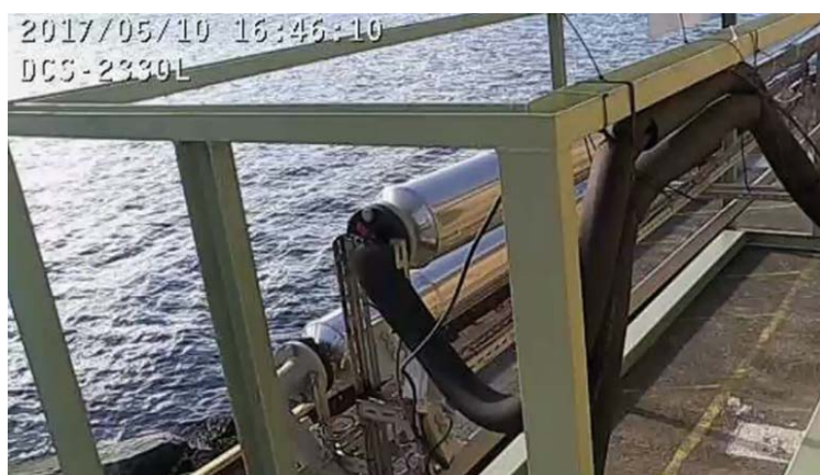
Fig 4(c) – Above: Layout of sensors and various pipeline segments (varying degrees of corrosion protection).
