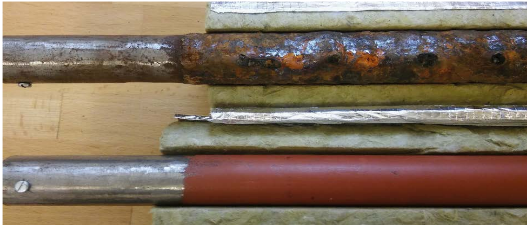
Fig 2 - Extension of the technique to measure CUI
