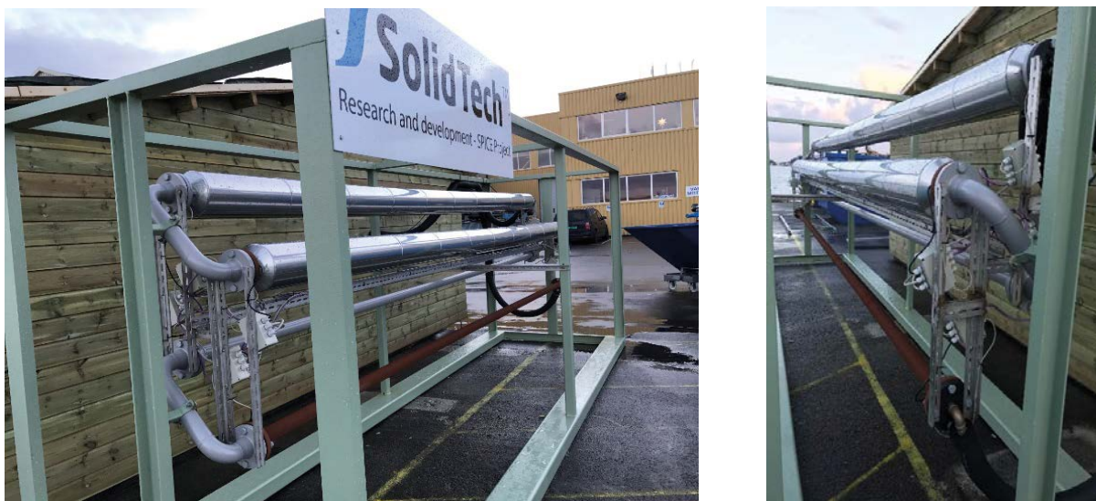
Fig 4(b) - Beta test rig on Location in Kristiansund, Norway. Pipeline covered with thermal insulation and cladding and continuously circulates hot water in a closed loop system. The EIS system is connected at convenient nodes and provides full real-time streaming telemetry back to UK control and monitoring centre.
